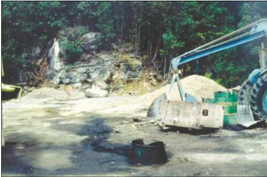
Figure 17a. Fuel oil spills can rapidly contaminate karst aquifers. (Photograph courtesy Elerly Hamilton-Smith.)
