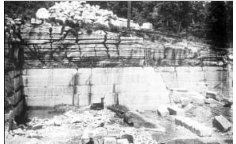
Figure 4. Dimension stone quarry showing weathered outcrop (top) and smooth working face of quarry. Vertical solution channels following fractures and joints in the weathered outcrop extend down into the smooth working face. Horizontal solution features occur between beds of the rock. Notice ladder for scale. (USGS photographic library - Loughlin 154.)
